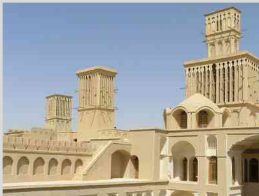
IR, Abarkuh, airing chimneys
